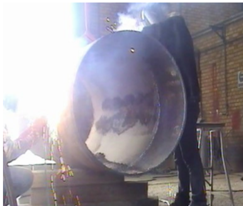
Fig. 1. Girth welding of the pipe.
