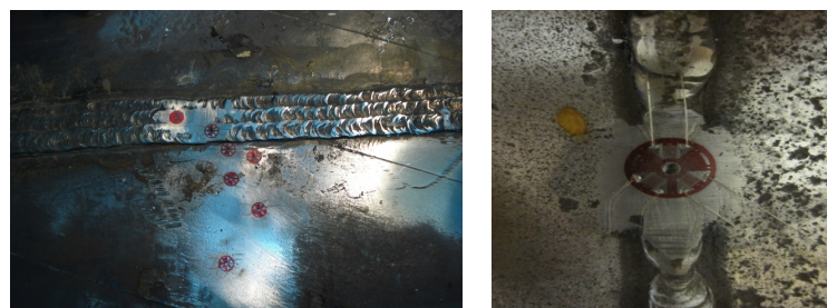
Fig. 2. Residual stresses on the external surface of the pipe.
